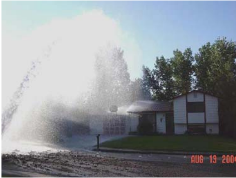
Figure 1. Failure of a pipeline in a residential neighborhood resulting in extensive damage to the house.
